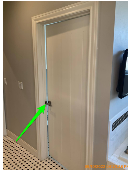
The master bathroom toilet room door did not latch properly
