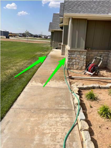
Head spraying against the wall at the front
