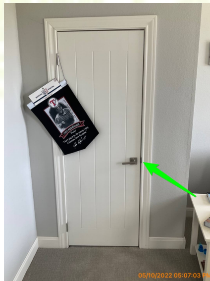
The front right bedroom closet door did not latch properly
