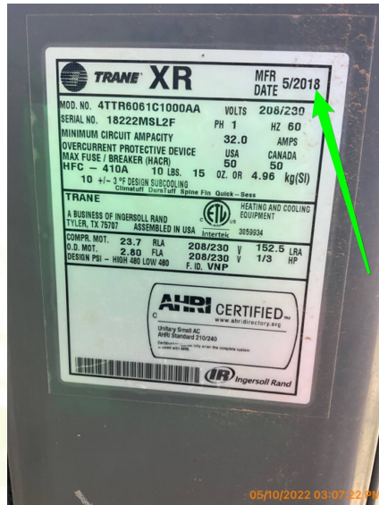
Trane condensing unit manufacturers data plate and date of manufacture
