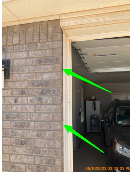
Areas needing sealed around the garage trim
