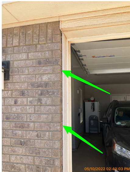
Areas needing sealed around the garage trim
