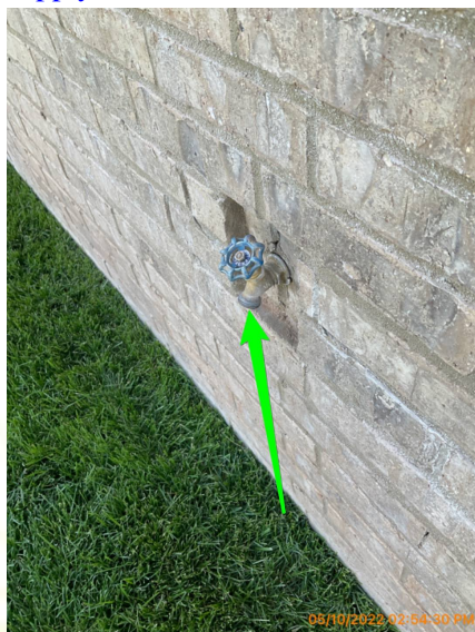
Missing anti siphon device at the rear exterior hose bibb
