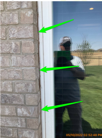
Areas needing re-sealed around some of the windows
