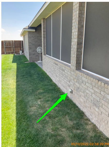
The rear exterior GFCI would not trip
